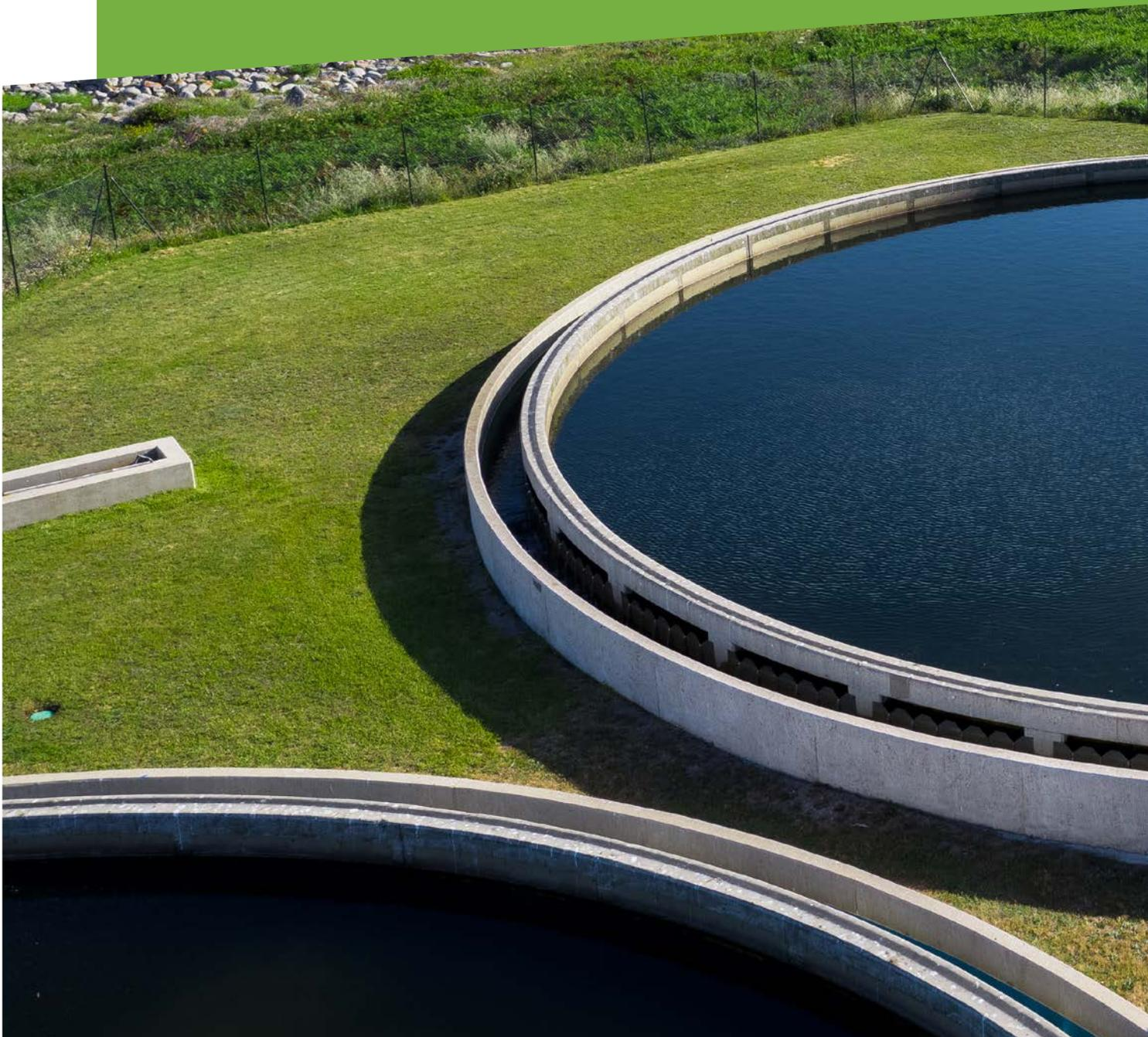
sical treatment plant to be purified and then conveyed into the municipal sewer network. Thanks to the new project, a portion of the purified industrial wastewater will be recovered and reused for washing the on-track machines. This water management system will allow the Catanzaro Workshop to save up to 80% of the water
